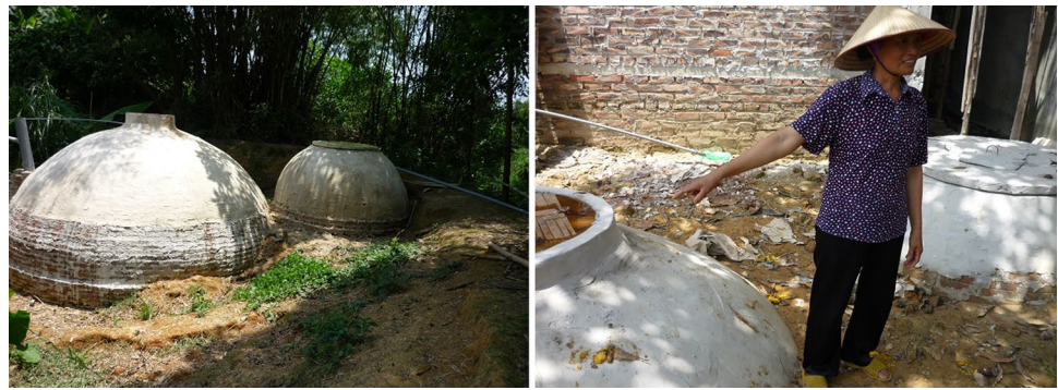
Fig. 1 The top of the biogas digester being built on Interviewee 4's land (left). Interviewee 3 showing her biogas digester (right). Source: Pictures taken by the authors
